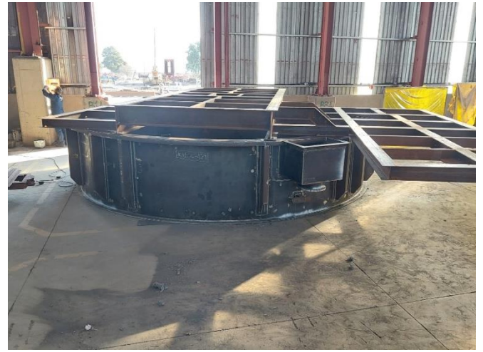
Figure 7: CIL Tank fabrication
