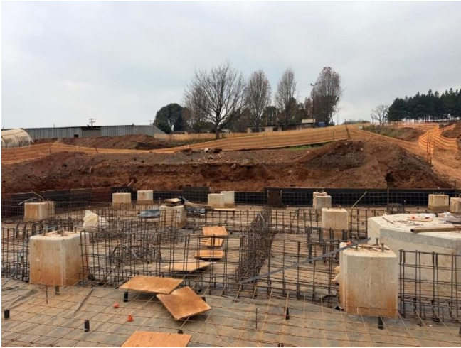
Figure 4: Elution circuit foundations
