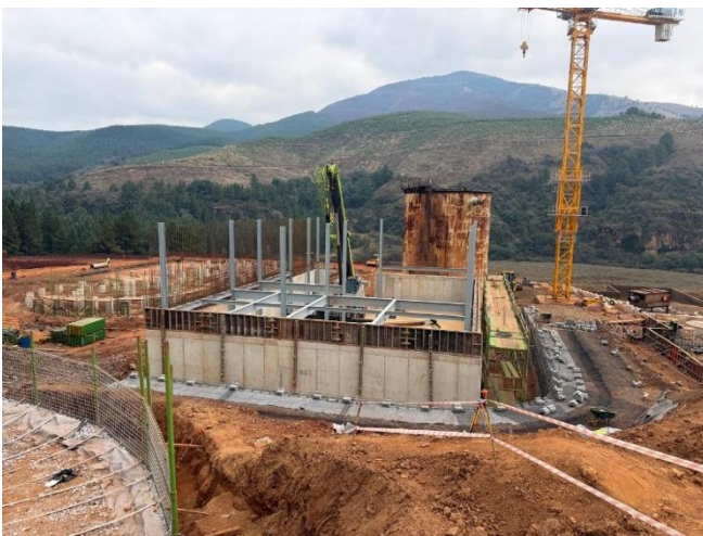
Figure 6: Gold Room construction continues - steel works
