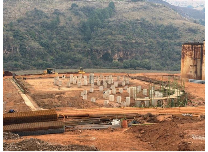
Figure 5: Thickener tank/processing area foundations
